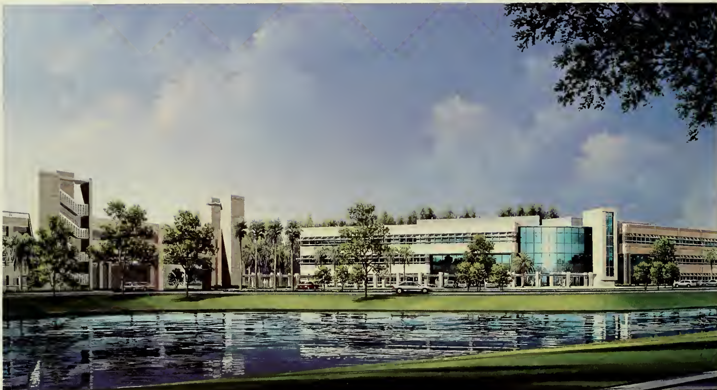
Architects: Hellmuth, Obata + Kassabaum, Inc., Tampa
